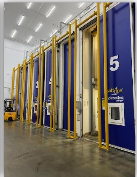
Soft Ripe Facility
